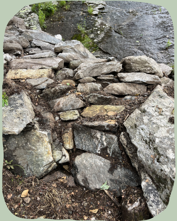
Retaining wall side view of east steps
