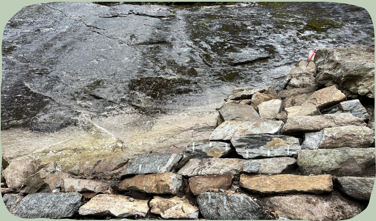
Retaining wall side view of the west steps
